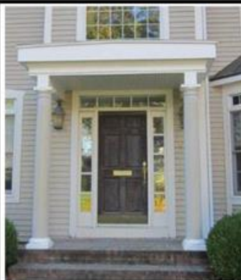
Maintenance-free Portico with fiberglass columns & Tuscan tops and bases
